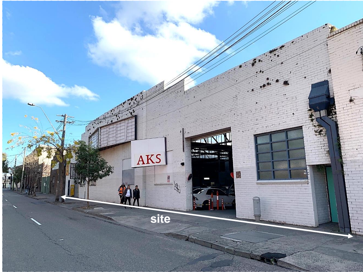
Botany Road frontage of site
