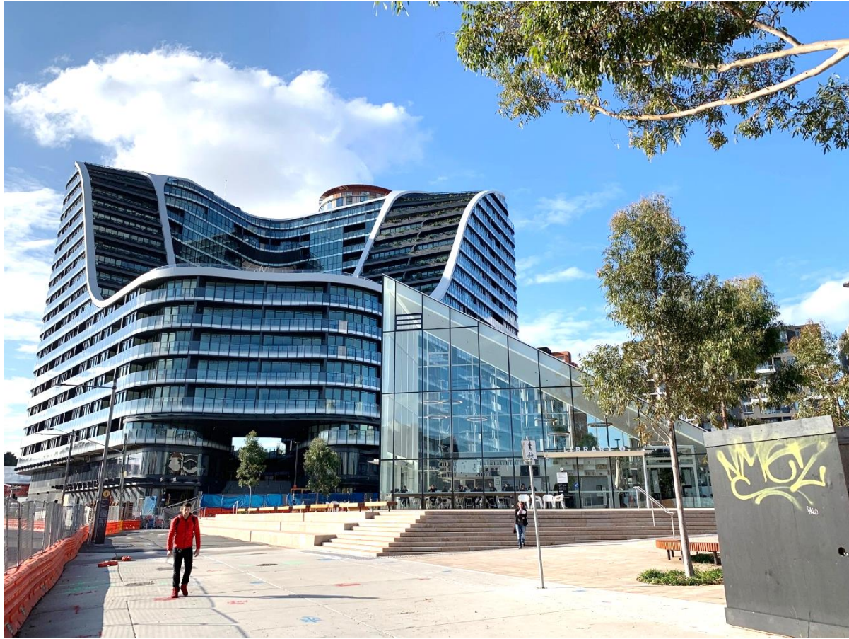
Green Square library and Infinity building
